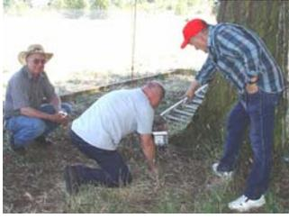
Drive the ground rod into the ground 2' out from the base of the tree leaving about 3' of the rod above ground level. Attach a short piece of rope to a egg insulator and attach the other end of the insulator to the copper wire so that the insulator/wire is about 6' above the top of the ground rod. Leave enough wire to connect to the tuner.
